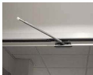
Closing regulator on double leaf door (standard)
