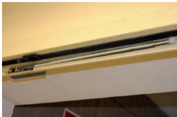
Closing regulator fire rated CE marked according to standard EN 1158 in closed position (left) and open (right)
